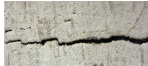
Lack of fusion
